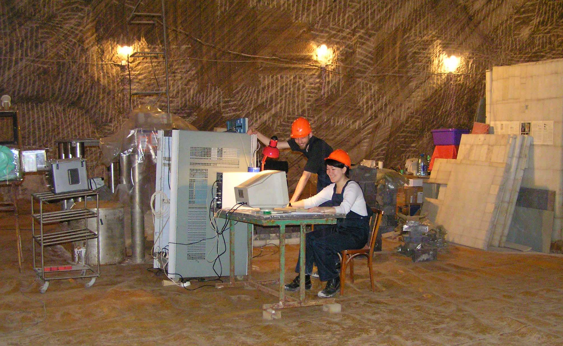
We plan to build a clean room of 10 000 class up to the end of 2006
